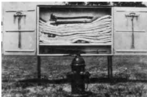
Figure A-2-6.2.4(c) This type of hose house can be installed on legs as shown or installed on a wall near, but not directly over, a private hydrant.
