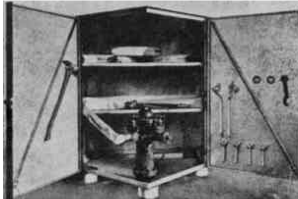
Figure A-2-6.2.4(a) House of five-sided design for installation over a private hydrant.
